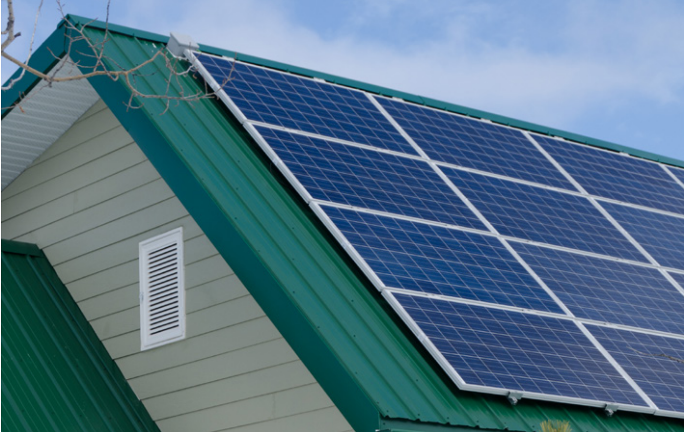
Home with solar panels.
